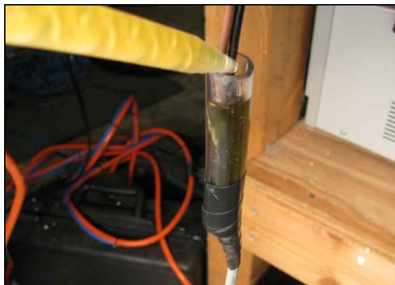
Figure 9: Squeeze Epoxy into the Vinyl Tube
