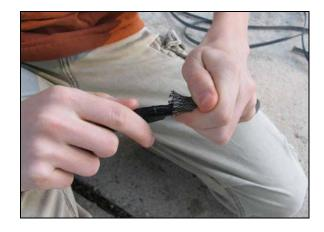
Figure 24: Feed Sleeving over the Cables
